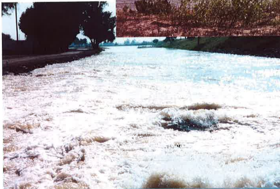
Rio Hondo Spreading Grounds , intake shown just downstream of the Parshall flume measuring station.
