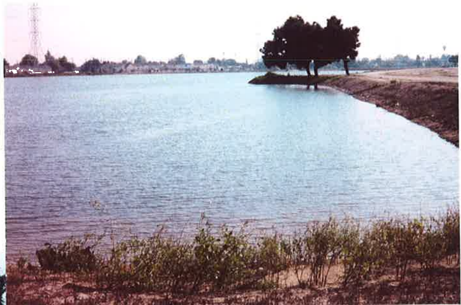
Rio Hondo Spreading Grounds , a percolation basin on the east side of the Rio Hondo Channel.
