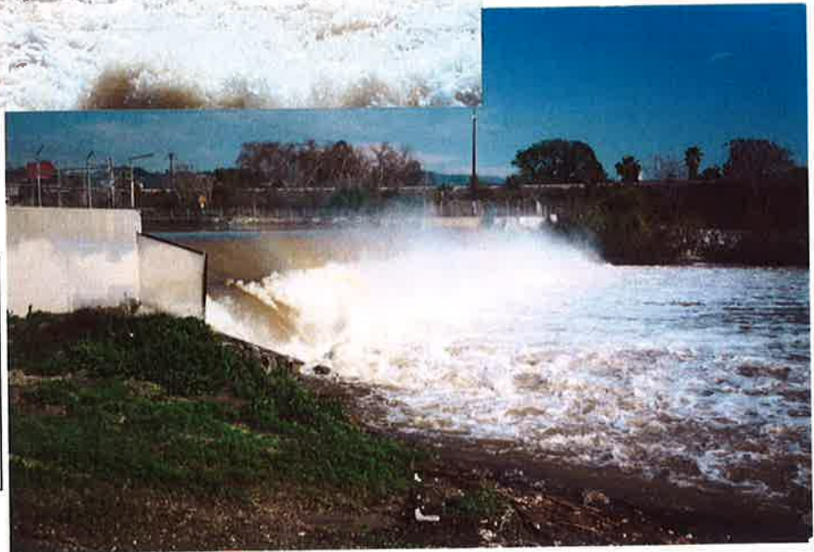
San Gabriel River , storm flows over rubber dams and drop structure. Rubber dams increase wetted area and infiltration.
